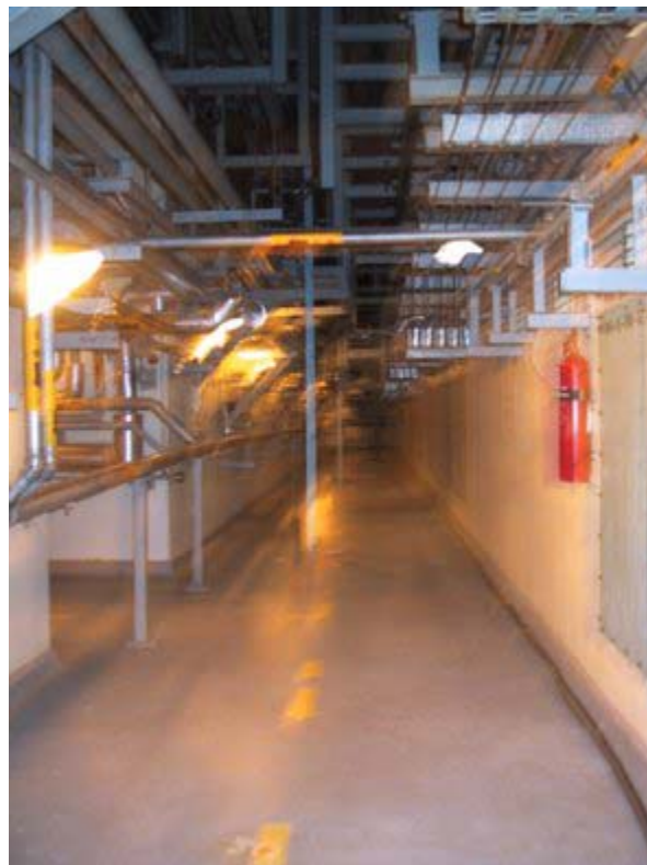
Fig 2 Valve Maintenance Access Area – Corridor EA51
